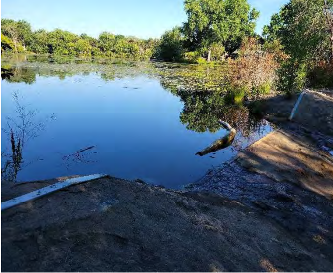
Photo #1: Grouted Weir, STA: 45+15
