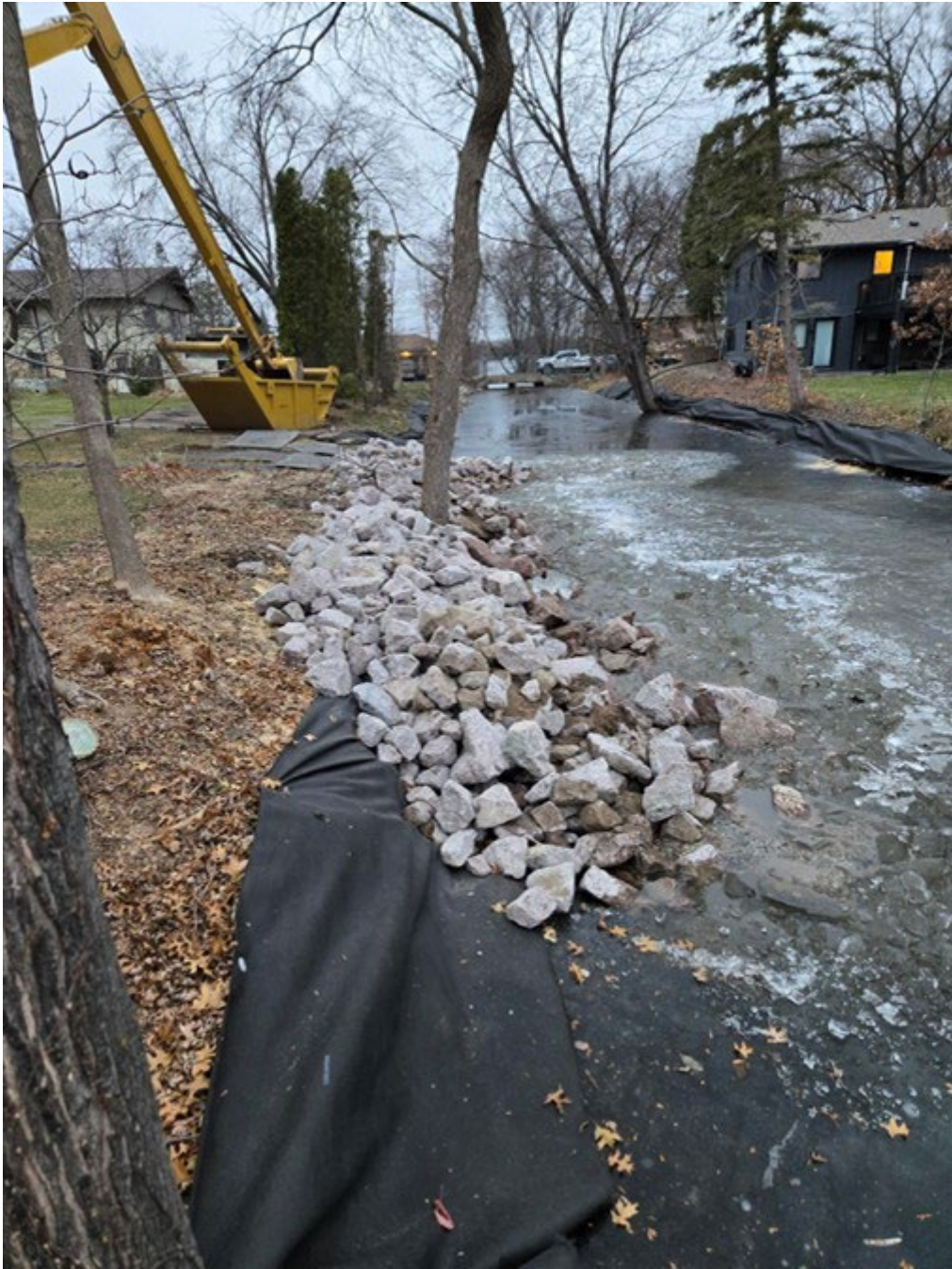
Riprap placement looking south to Little Lake Johanna
