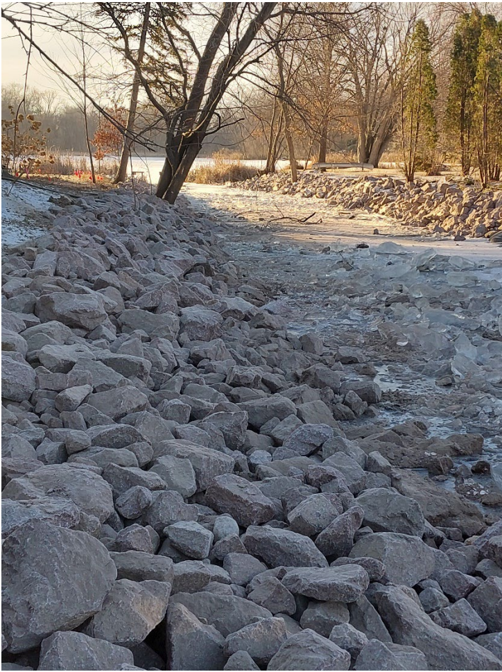
Placed Riprap Looking south to Little Lake Johanna.
