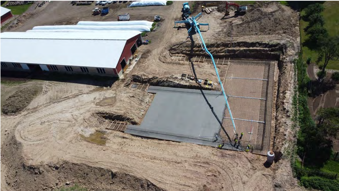
Figure 9 Floor concrete pour, QA mix, times, temperature, and placement Krcmarik 6/10/24
