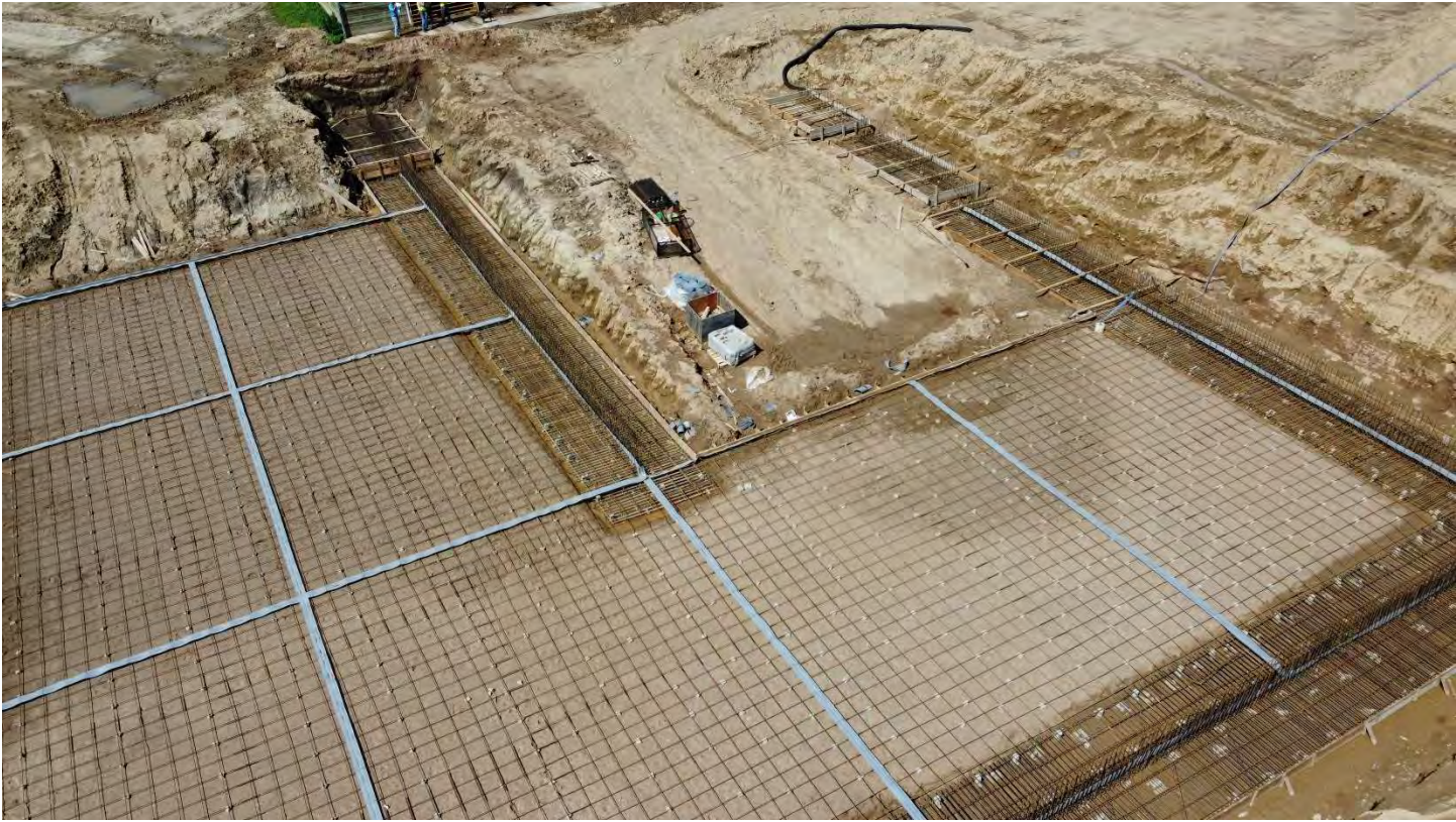
Figure 6 Steel and waterstop check, Krcmarik 6/4/24
