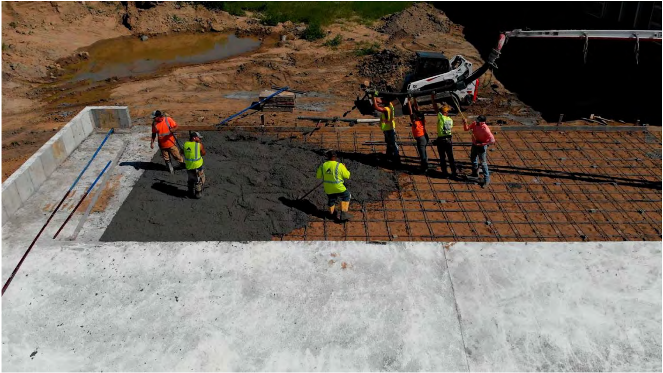
Figure 17 Apron placement, Krcmarik
