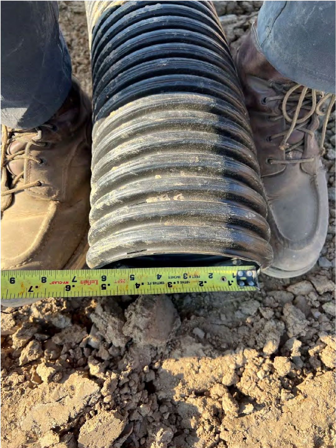
Figure 4 Tile material and size check, 5/13/24
