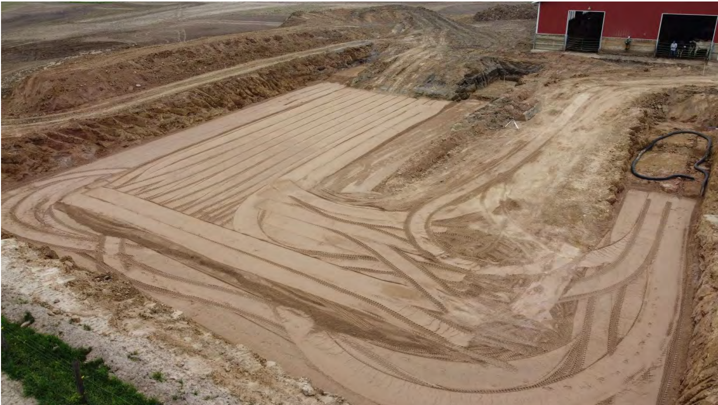
Figure 5 Sand base depth and compaction check, Krcmarik 5/15/24
