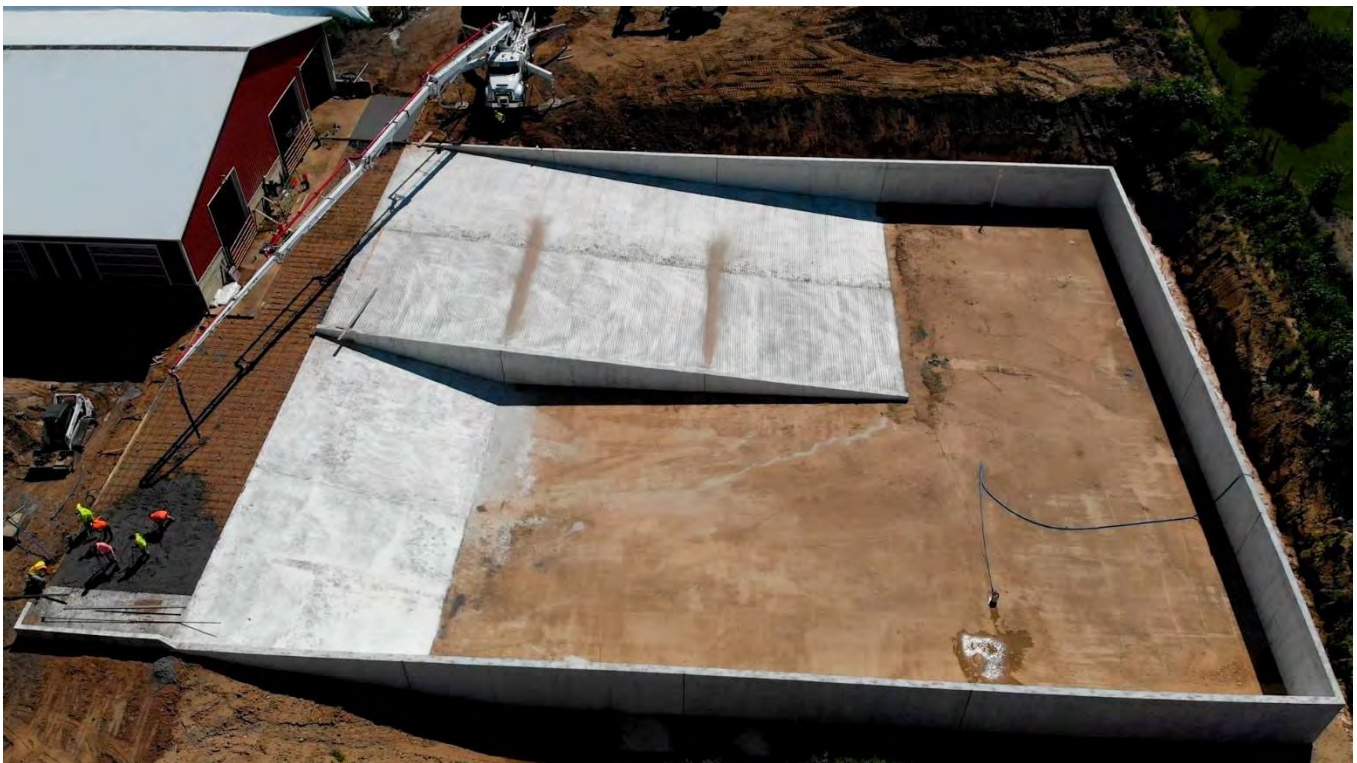
Figure 16 Ramps cured and apron placement underway, Krcmarik
