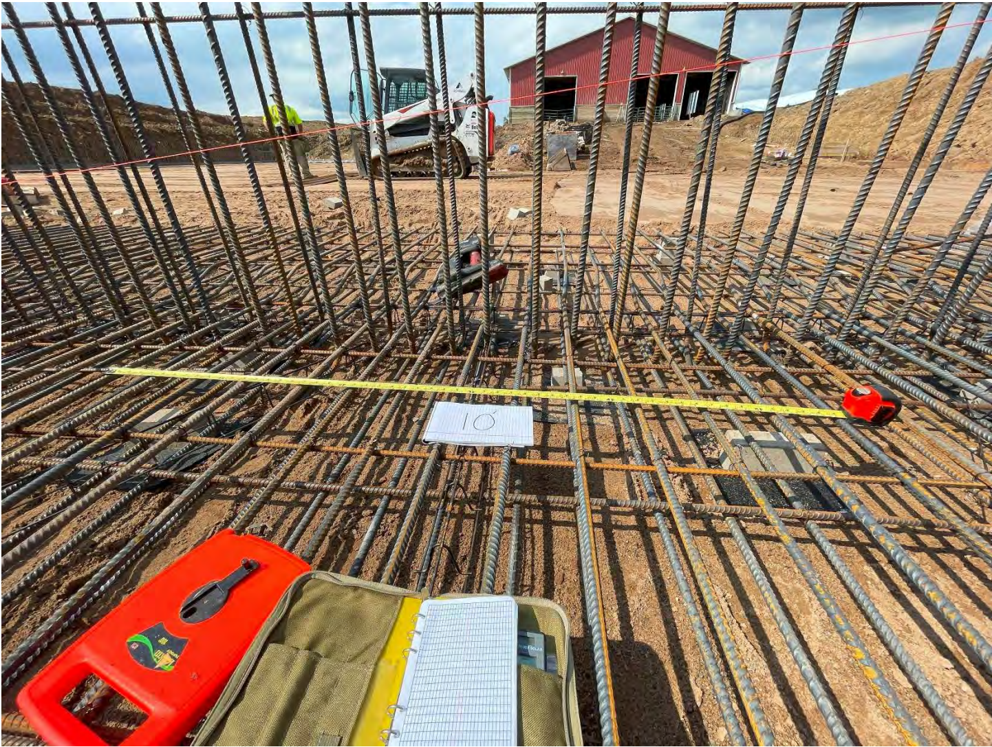
Figure 7 Steel bar spacing, size, and clear check, Krcmarik 5/24/24
