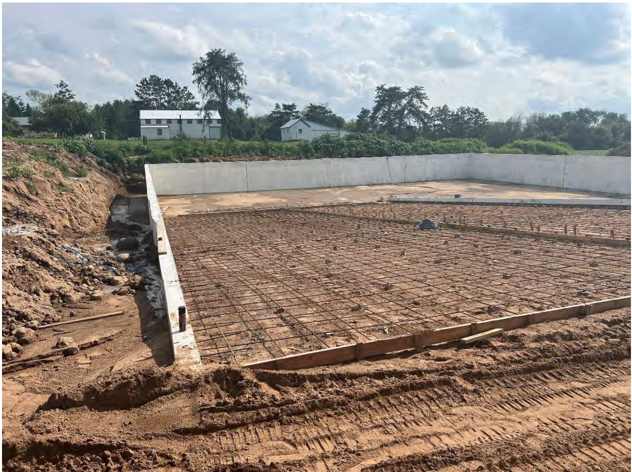
Figure 14 Ramp steel before placement, Krcmarik
