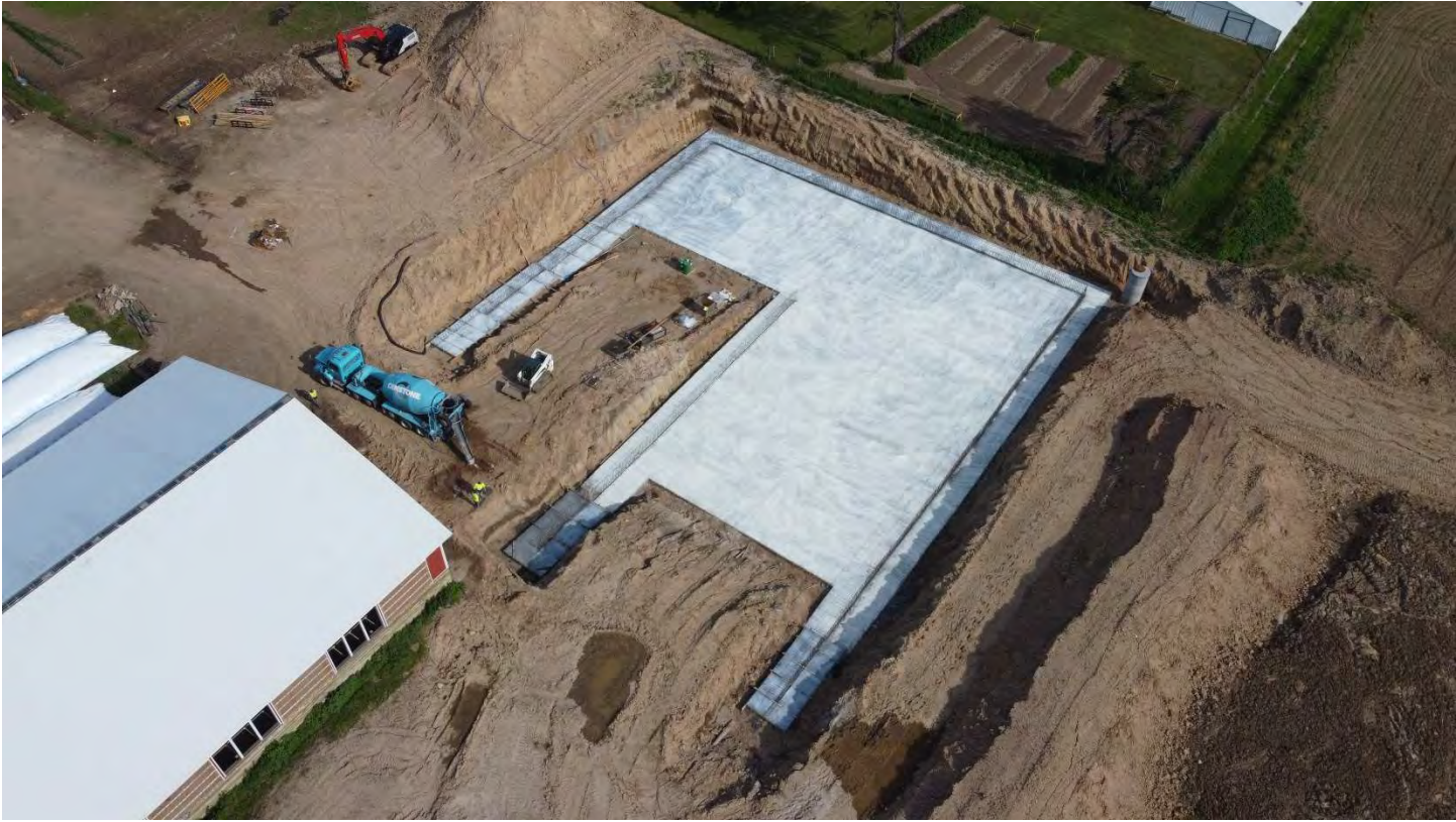
Figure 10 Floor concrete sealed and saw cut, Krcmarik 6/10/24
