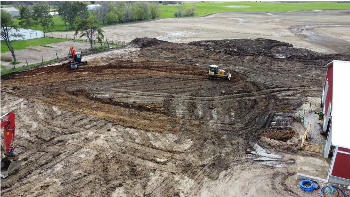
Figure 1 Topsoil and organics stripped, fence and watering facility removed, Krcmarik, 5/1/24
