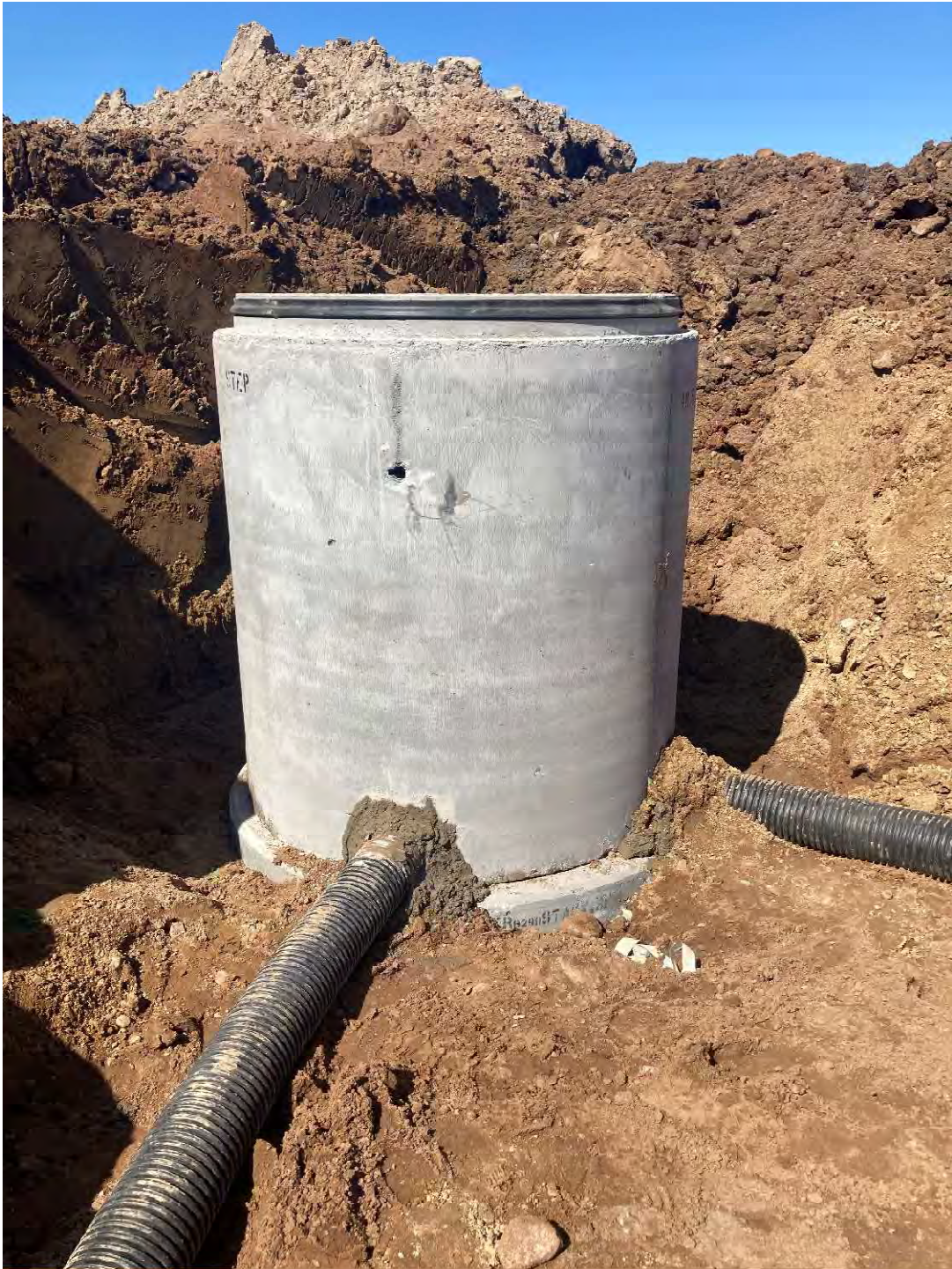
Figure 3 Catch basin well elevation, size, precast stamp, and seal check
