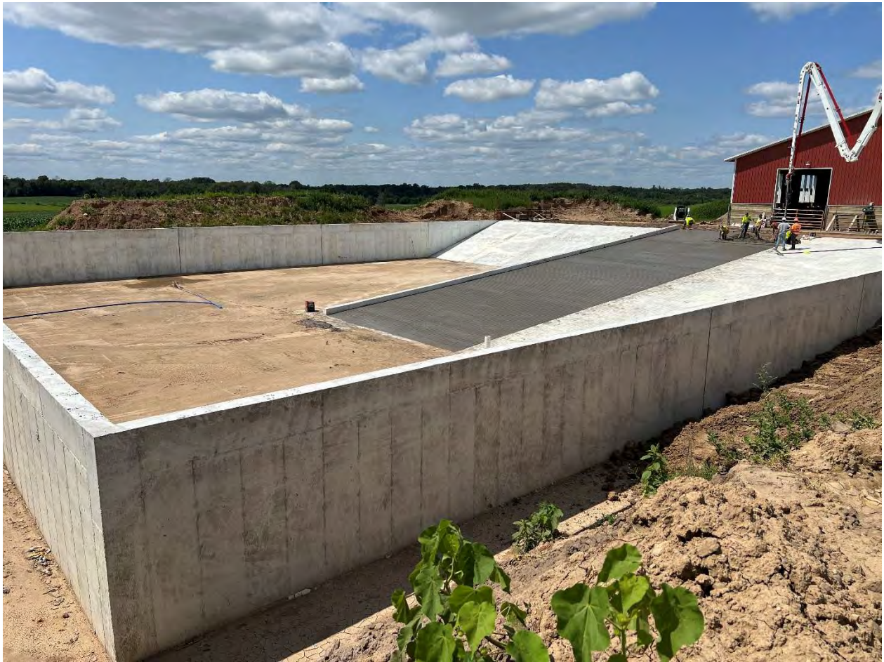
Figure 15 Final Ramp, placement Krcmarik
