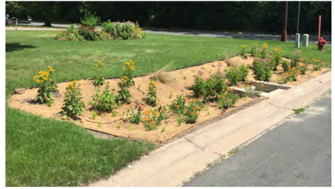
Recently installed rain garden
