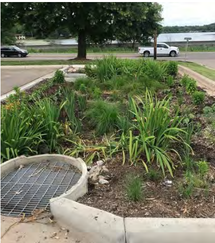
Completed rain garden in Shoreview
