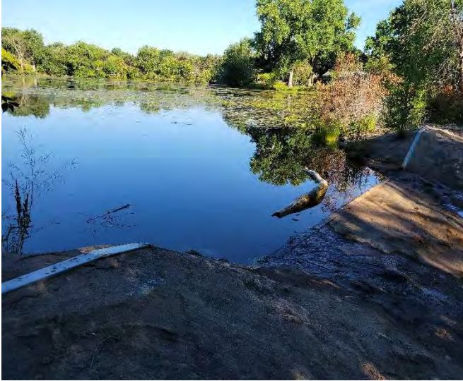
Photo #1: Grouted Weir, STA: 45+15
