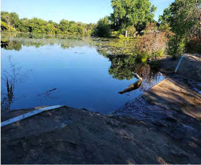
Photo #1: Grouted Weir, STA: 45+15
