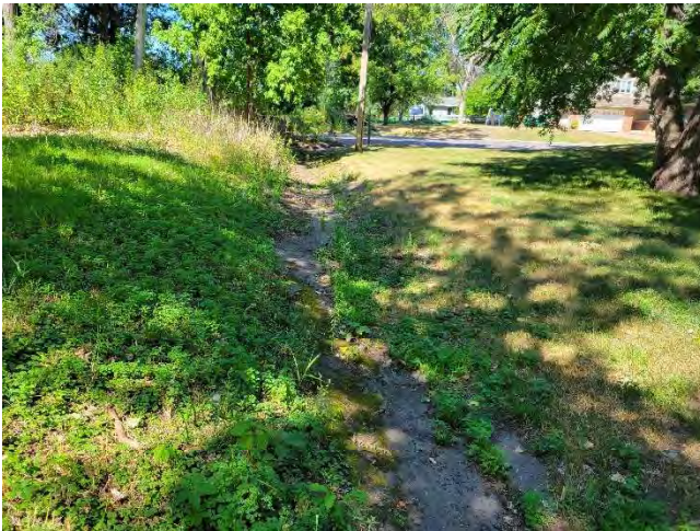
Photo #3: Swale on west side of ditch, STA: 42+00
