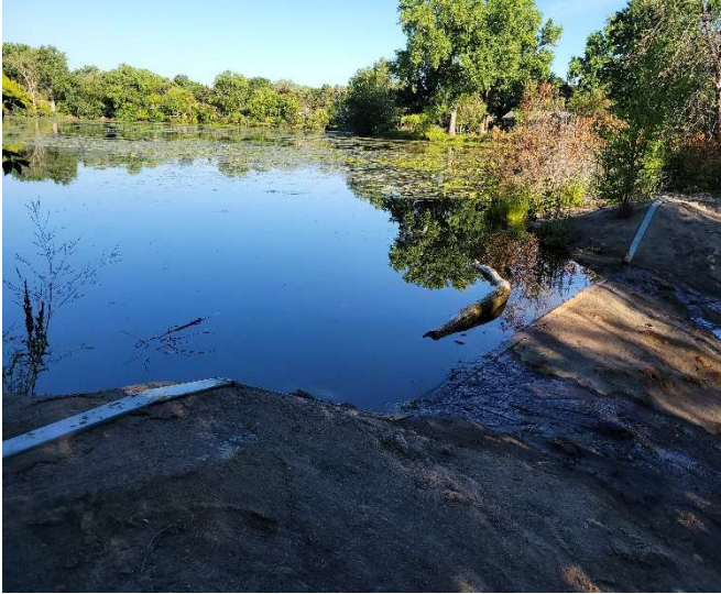
Photo #1: Grouted Weir, STA: 45+15
