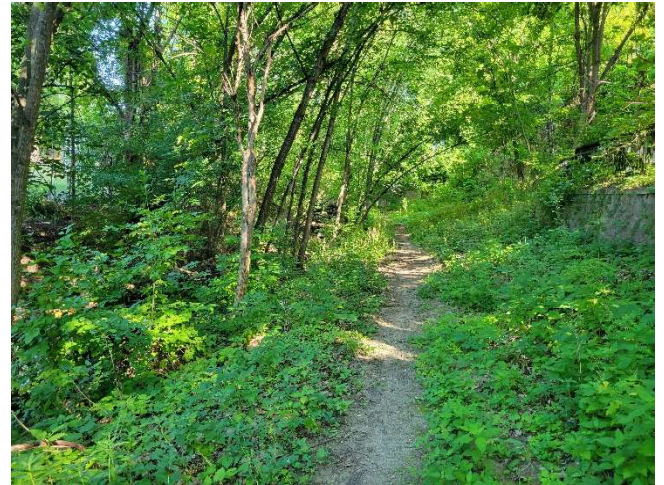
Photo #4: Gravel Path and Retaining wall on east side of ditch, STA: 30+00
